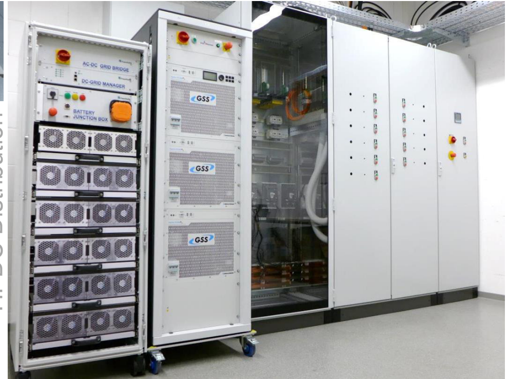
Main bus bar with currents up to 1600 A and a bipolar 380 V DC voltage
